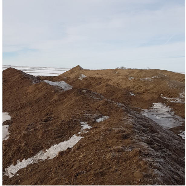
6. Dirt pile – Km 159+325 – Nov 25, 2017
