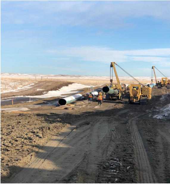
1. Bending crew – km 160+000 – Nov 24, 2017
