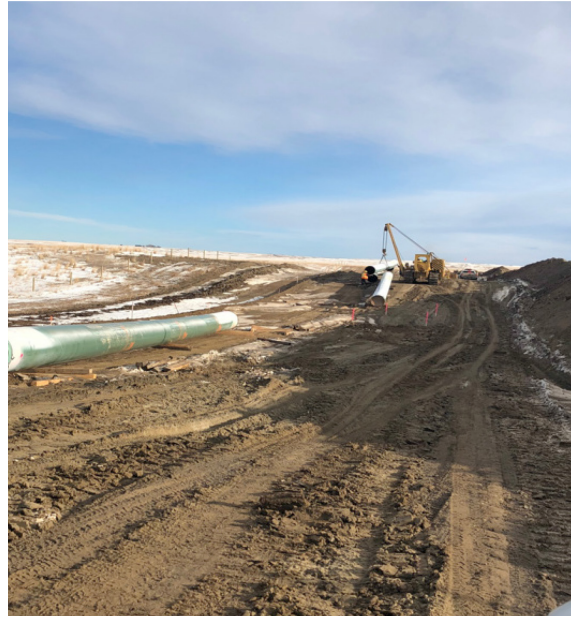
2. Bending Crew (East) – Km 160+000 – Nov 24, 2017
