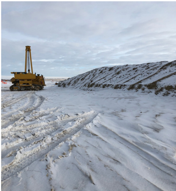
3. Transition Soil (S.E.) – km 159+350 – Nov 25, 2017
