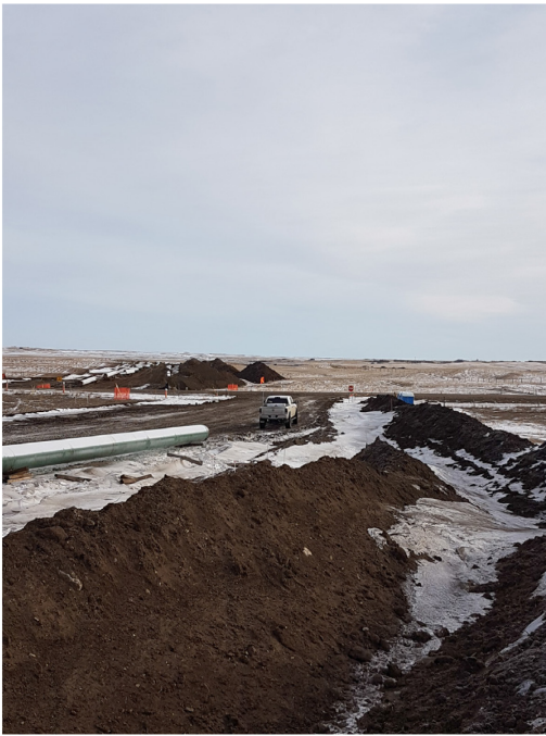
7. Dirt Pile (West) – Km 159+325 – Nov 25, 2017
