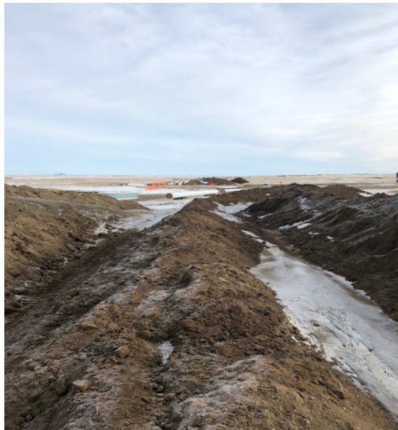
4. Transition pile (East) – Km 159+350 – Nov 25, 2017
